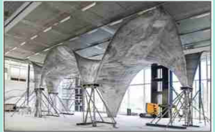
Fig 1 Ultra-thin curved roof using novel formwork system
